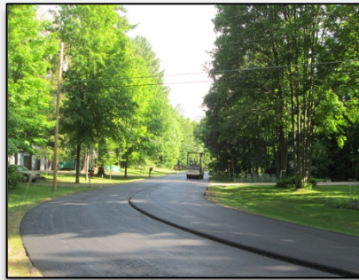
Subdivision road resurfacing project
