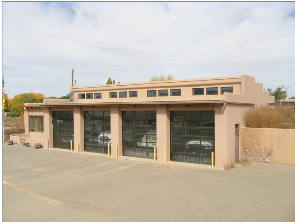
Galisteo Fire Station
