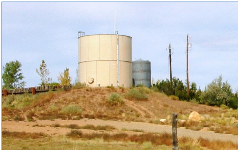
Galisteo Water Tank
