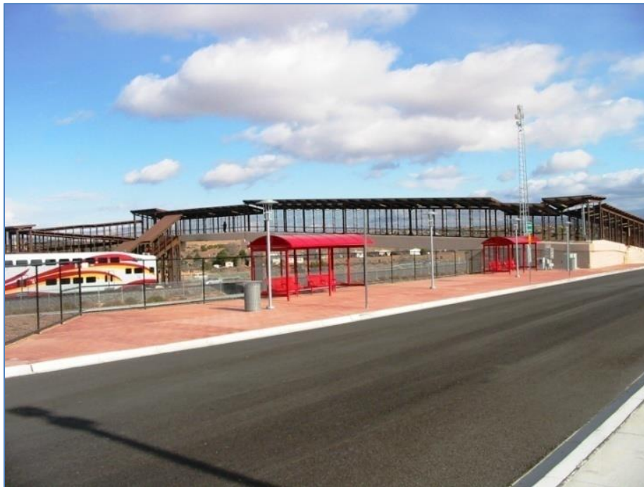
Rail Runner Station at NM 599
