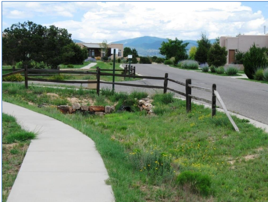
Example of Low Impact Stormwater Management Using Vegetation and Swales
