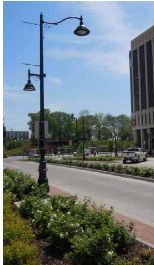
Improvements at 7 th and Minnesota Avenue
