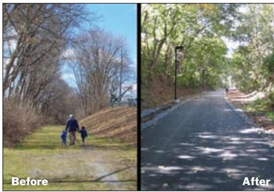
Converting abandoned rail lines like this one in Ephrata Borough provides recreation for residents as well as an alternative means of travel.
