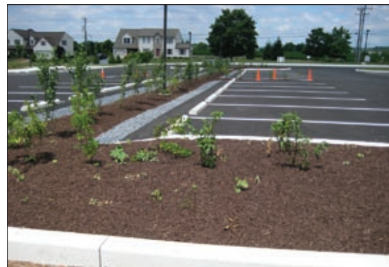
Incorporating green infrastructure interventions such as these biofilters at the Warwick Township Municipal Office, into traditional capital improvement projects can be an effective means of improving the quality of storm water runoff.
