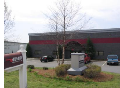
According to the market assessment, the Central Area will be able to support an additional 400,000 to 500,000 square feet of office space.
