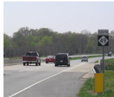
Among the major roadways that serve the Central Area are US 601, NC 73 and NC 49 (shown above).
